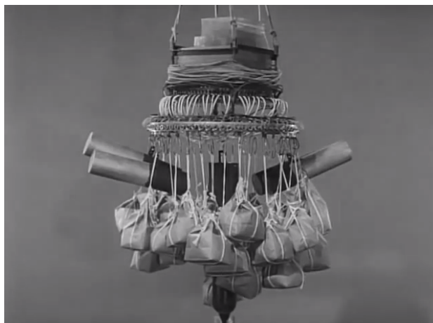
Figure 5. A close-up of the sand bags used to ballast the balloons. Sand bags would drop if the balloon was too low in the Jet Stream, and hydrogen would release if it was too high (Sacchi and Nicosia, 2013).
